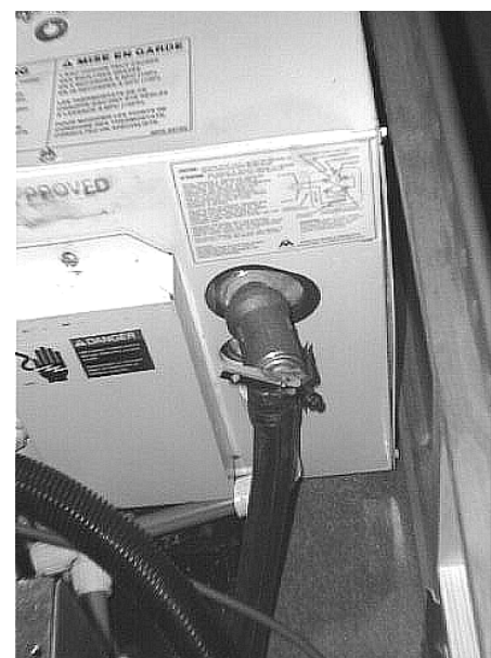
Pressure-Temperature Relief (P-T) Valve
