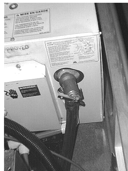
Pressure-Temperature Relief (P-T) Valve
