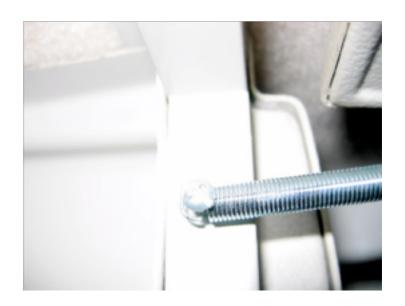
Notice that on the cabinet door inside there is a ridge that sticks out. Your pilot hole should be on the outside of this ridge. Sight very carefully the line between the screw in the frame and the screw location in the cabinet door.
