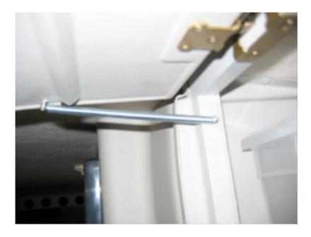
Drill a very small pilot hole on the inside of the side cabinet frame, about 1" down from the top of the frame, and centered side to side in the wood.
