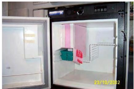
Freezer with door open. Two full-sized ice trays ( $4\ 1/4" \times 10\ 3/4"$  with 14 cavities) fit nicely and freeze ice cubes overnight. Note: Although not obvious, the side panel does not go to the back wall, but instead, an aft panel fits between the aft fins of the cooling section, so the temperature sensor remains in the refrigerator compartment and not in the "Super Freezer" compartment. Also, the lower forward part is trimmed so as not to interfere with pop cans in the refrigerator door.
