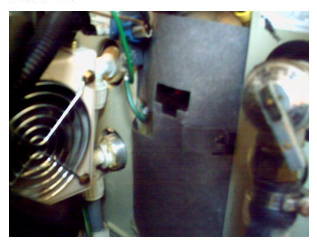
You may see a hard fiber board cover (this may be missing along with the bottom screw if the heater has ever been worked on). This cover may be held on with two nuts. These nuts are 10mm and should be easily removed. Once they are off pry the cover off. It goes behind the sheet metal cabinet just a little (don't worry if it breaks in two you can still use it).
