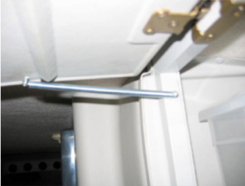
Drill a very small pilot hole on the inside of the side cabinet frame, about 1" down from the top of the frame, and centered side to side in the wood.
